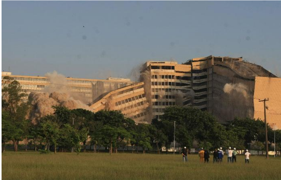
Figure 2.17: Demolition of hospital section, Ilha do Fundão, Rio de Janeiro, Brazil.
