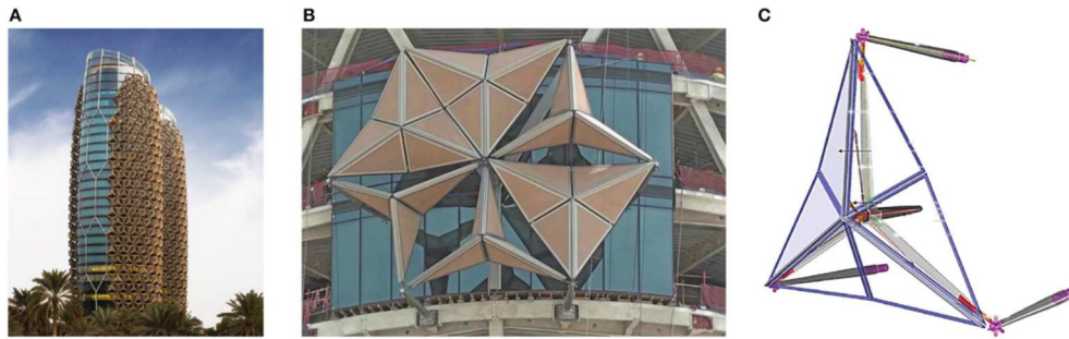
Figure 2.1: (A) Illustration of the Al Bahar towers in Abu Dhabi. (B) detail of a module of the ABS (picture taken during the mounting of the screens). (C) ABS actuation mechanism (reproduced with permission from Karanouh and Kerber, 2015).
