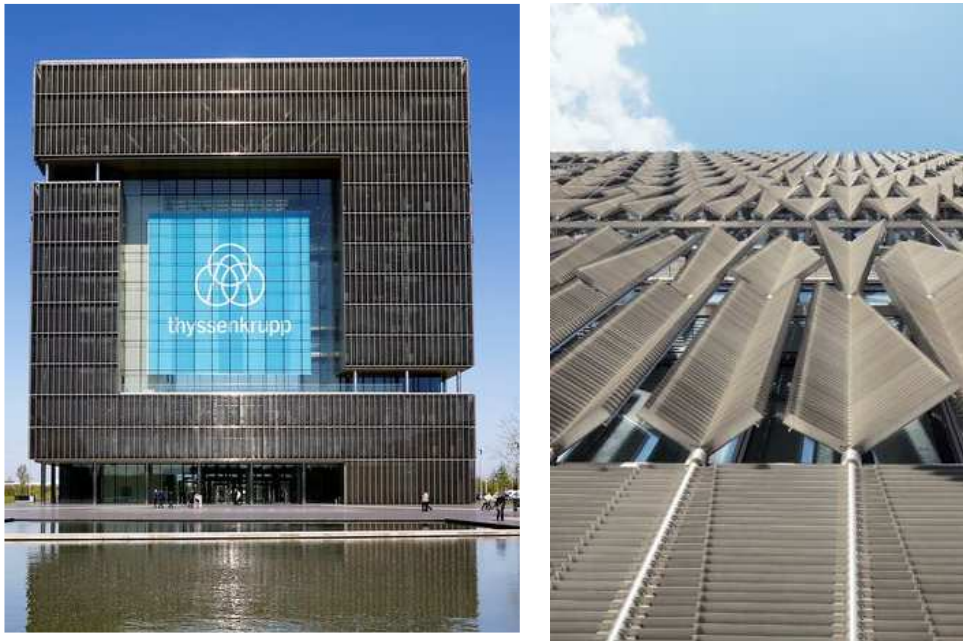
Figure 1.6: ThyssenKrupp Quarter Essen Q1 building – outdoor view.
