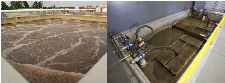
Figure 1-5 - Differences in color and viscosity in CAS (left) and MBR (right) oxidized liquor
