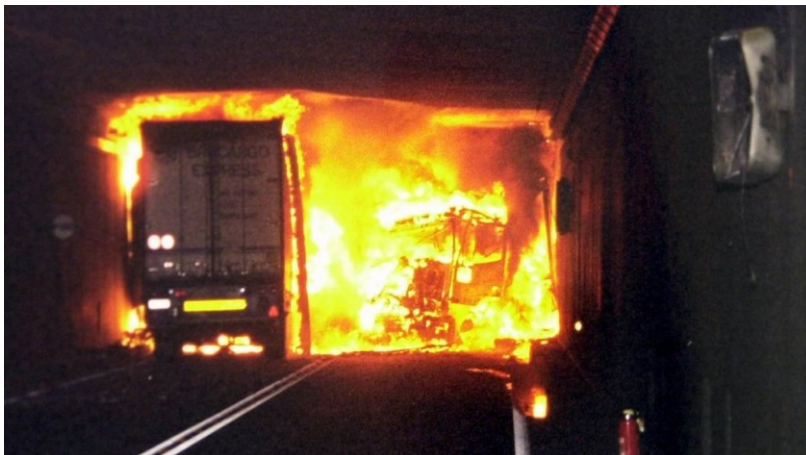
Fig. 1.3. Saint Gotthard tunnel fire in 2001 with 11 depths.
