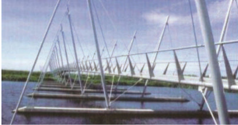
Figure 1.8: Bridge in Purmerend. Source: (Boeck, 2013, p. 19, [1]).
