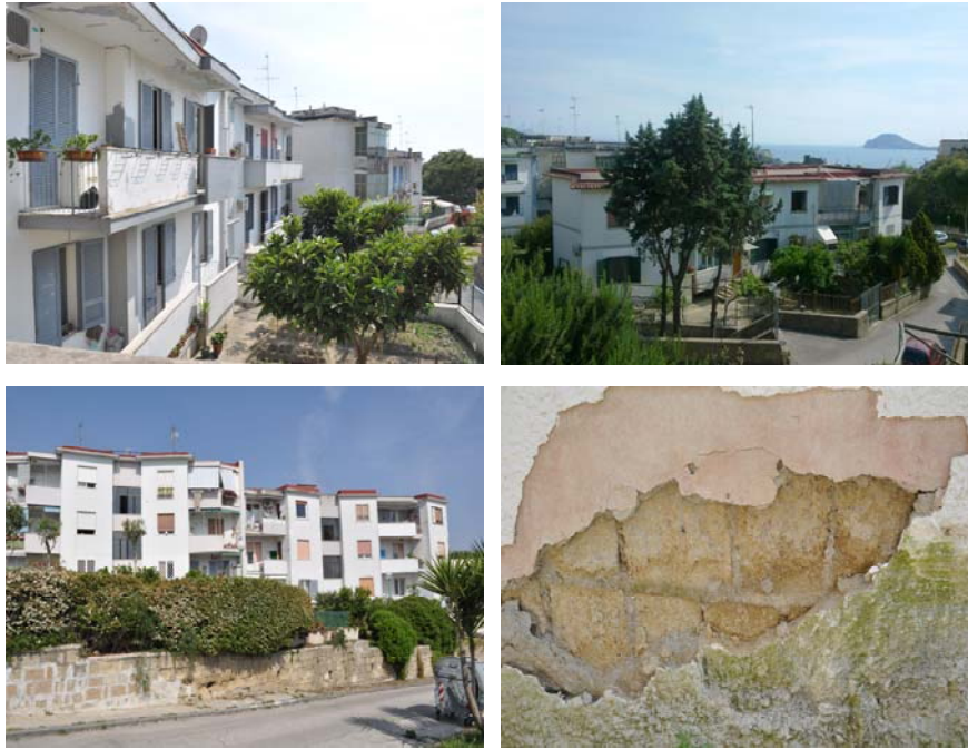
Fig. 5. 6: Quartiere INA-Olivetti, Pozzuoli (NA). Today. Tuff walls under the plaster
