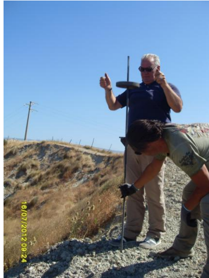
Figure 5.2 In situ investigations with steel bar.
