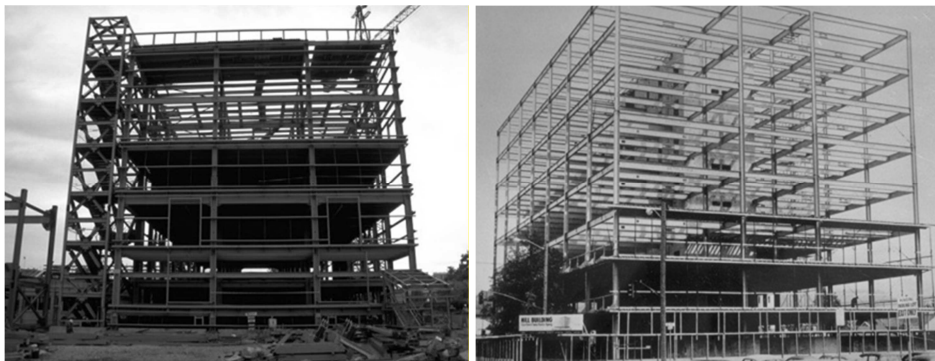
Fig. 2.1 – Steel Moment Resisting Frames in U.S.A.
