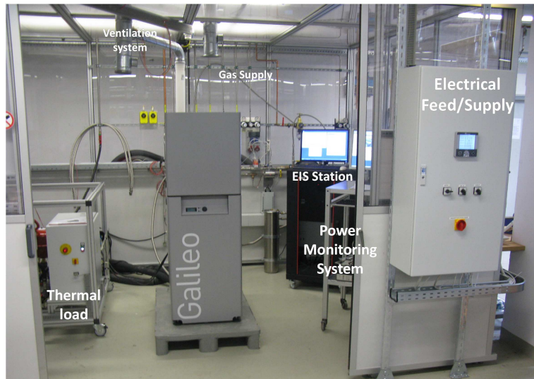
Figure 4.3 Picture of the EIFER test bench dedicated to the Galileo 1000N system testing [53].
