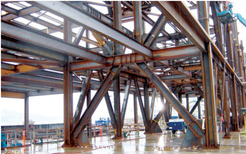
Figure 1.3 – EBFs with K-scheme made by double-T sections
