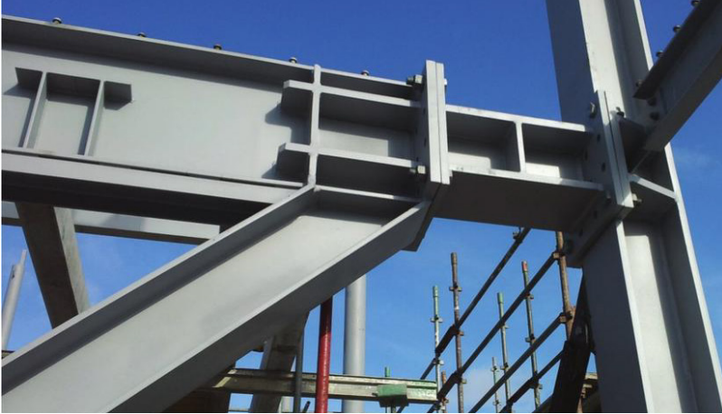
Figure 1.2 – EBFs with D-scheme made by double-T sections and removable link
