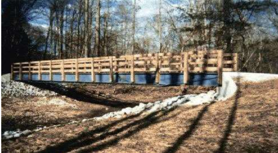
Figure 3. The Composite "Clear Creek" Bridge in U.S.A.
