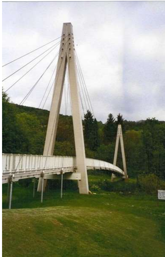
Figure 5. The Composite “Aberfeldy Bridge” Bridge in Scotland, U.K.
