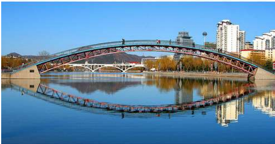
Figure 1. The Composite “Miyun Bridge” in Beijing, China.
