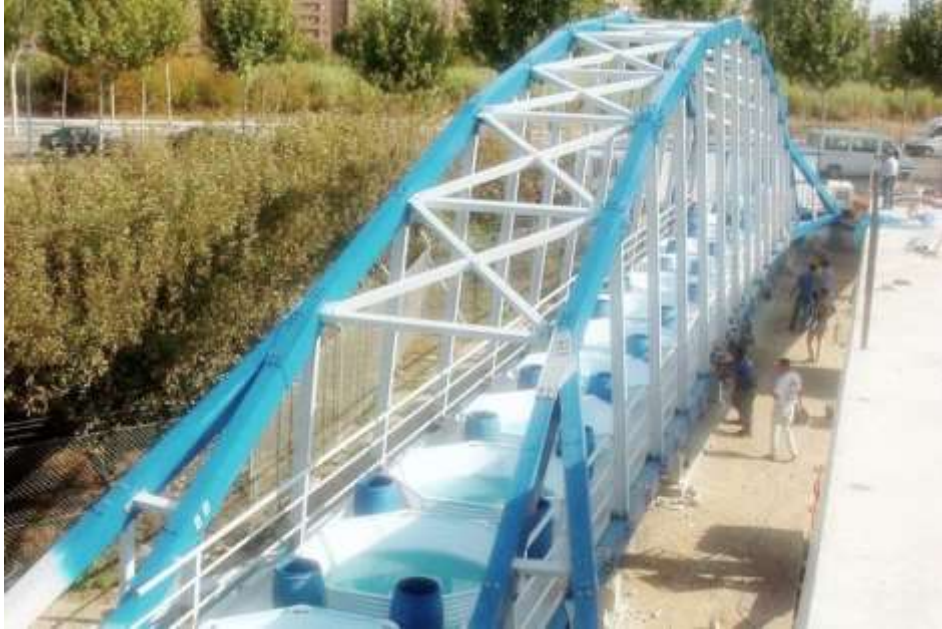
Figure 9. Lleida Footbridge in Spain.
