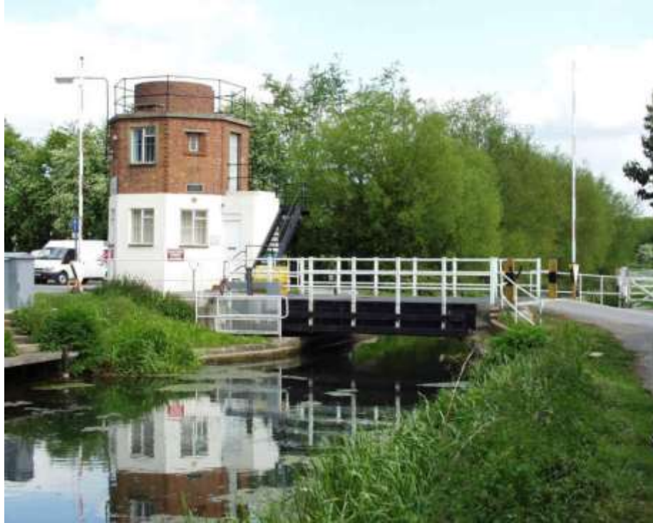
Figure 6. The Composite “Bonds Mill Lift” Bridge in Gloucestershire, U.K.
