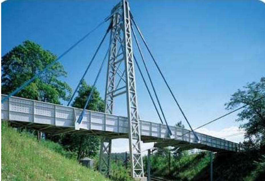
Figure 7. The Fiberline All-Pultruded Composites Cable Stayed; Kolding, Denmark.
