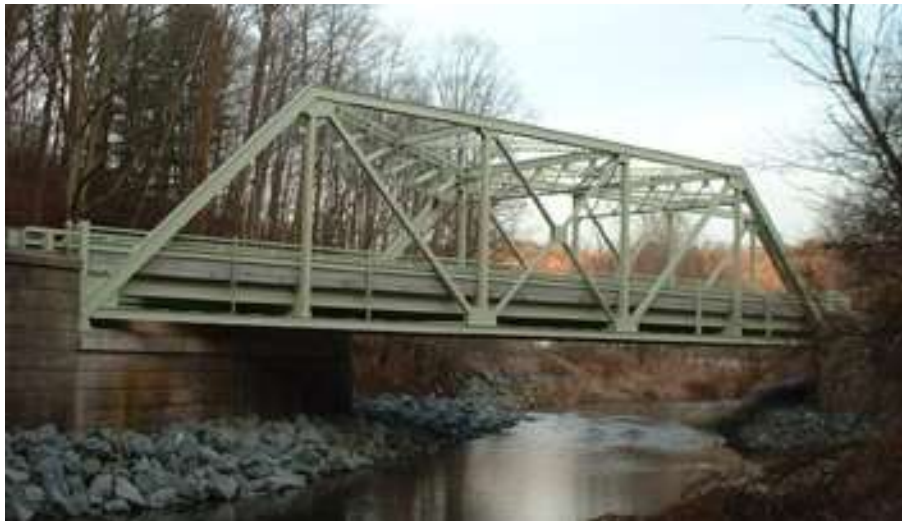
Figure 4. The bridge over Deer Creek; Maryland State, U.S.A.
