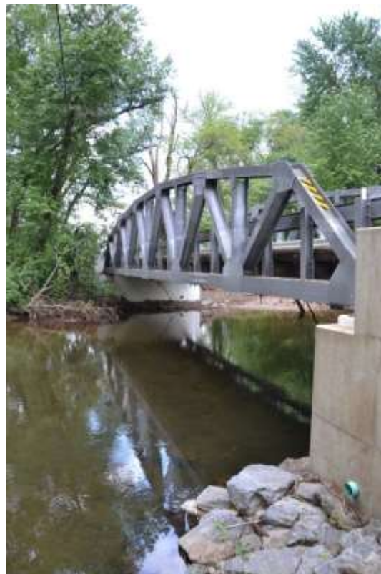
Figure 2. The Composite “Tom’s Creek” Bridge in U.S.A.
