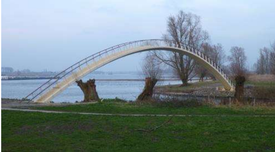
Figure 8. The Composite “Ooypoort” pedestrian Bridge in Nijmegen, Netherlands.
