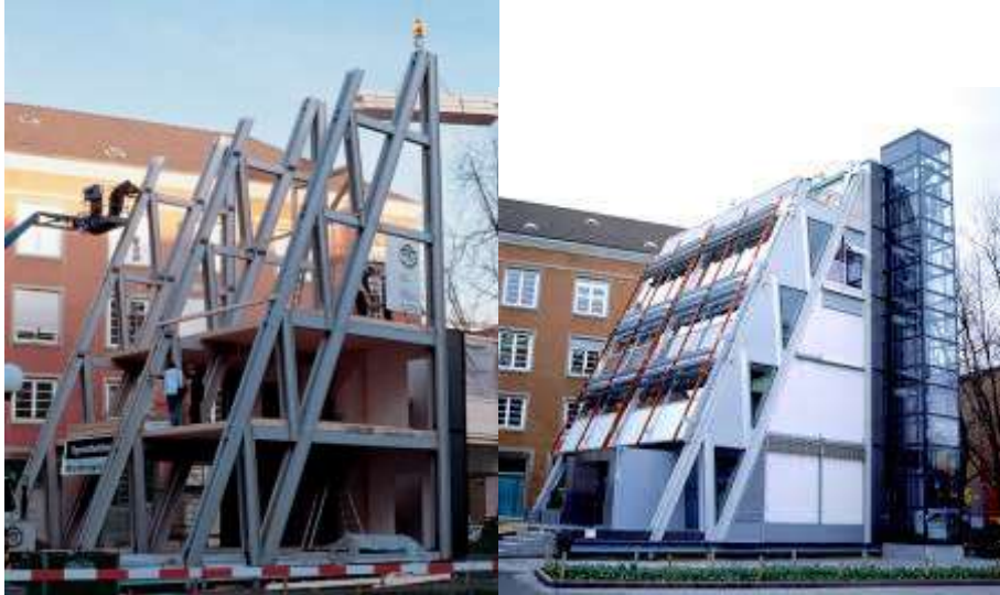
Figure 10. The All-Composite “Eyecatcher” Building in Switzerland.
