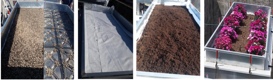
Figure 5.3 Drainage layer with clay and commercial panel filled with clay.
