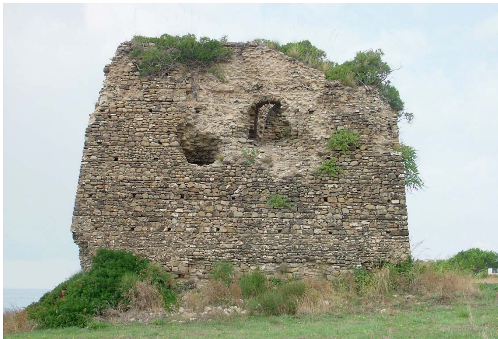
Figure 1.12: Torre Caleo, it is possible to see the use of larger stones at the base and the presence of rounded shape river
