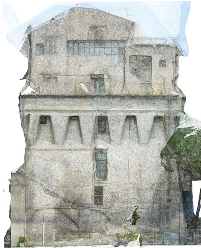
Figure 6.8: Ortophoto of the South-Est elevation of Torre di Vietri with Recap Photo
