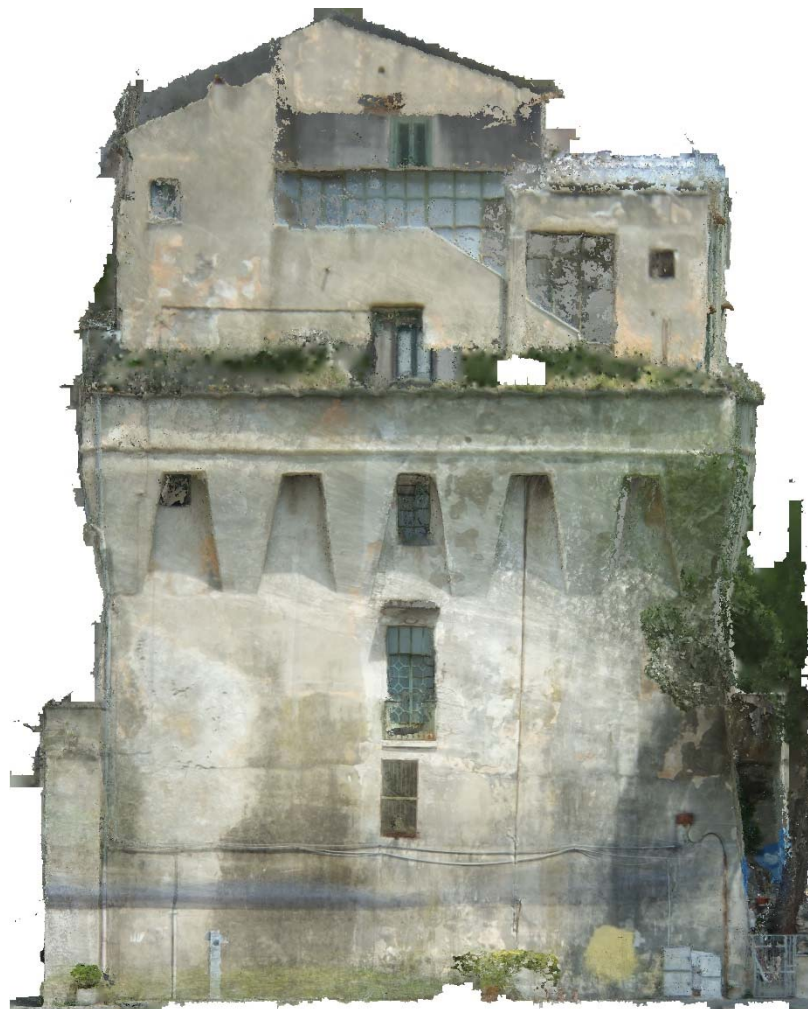
Figure 6.6: Ortophoto of the South-Est elevation of Torre di Vietri with PhotoScan
