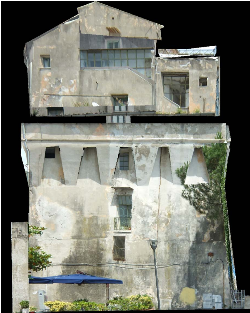
Figure 6.13: Ortophoto of the South-Est elevation of Torre di Vietri with Photo Modeller
