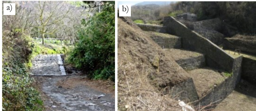
Figure 3.5 Examples of a) artificial reverbed channel and b) brindle with 4 steps realized during the XIX century (Cibelli, 2014).
