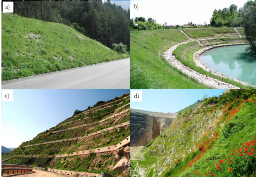
Figure 5.4 Examples of Prati Armati technology on a) road embankment, b) streambank, c) dam and d) calcareous cave applied in Italy ( www.pratiarmati.it ).
