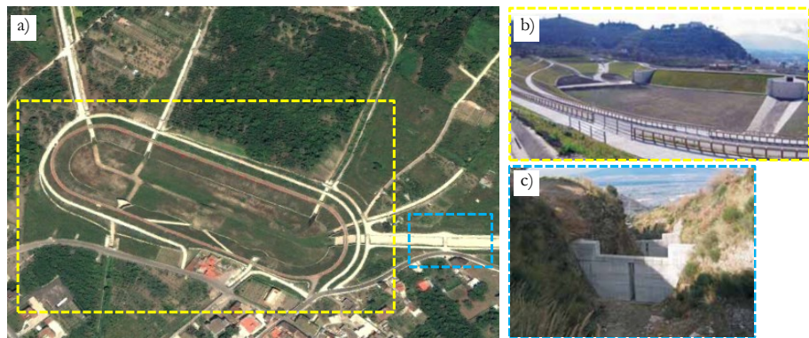
Figure 3.6 a) view from top of the dissipation basin at piedmont of Pizzo d'Alvano (where the May 1998 debris flows occurred) and particular of the b) dissipation basin and c) brindle.
