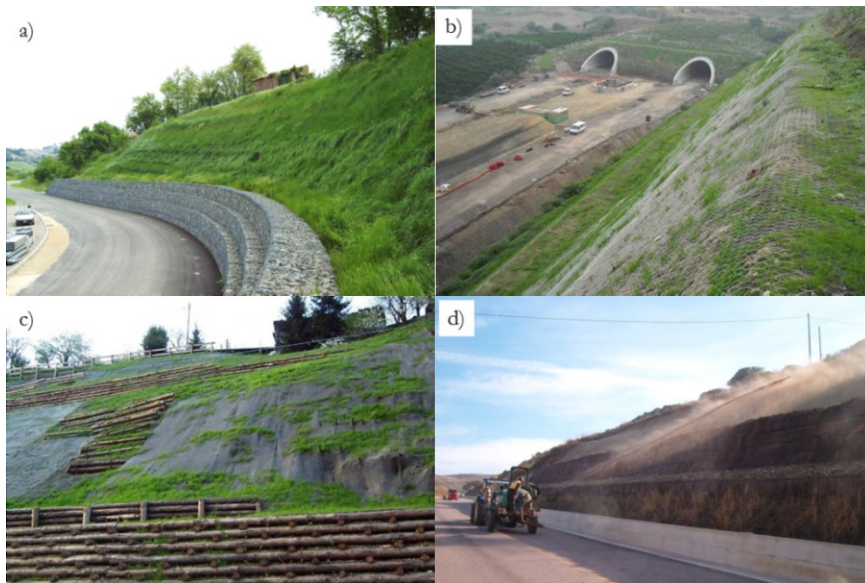
Figure 5.5 Examples of combined Prati Armati technology and active control works such as a) gabions, b) erosion control mat, c) woody fences and d) reinforced soil applied in Italy ( www.pratiarmati.it ).
