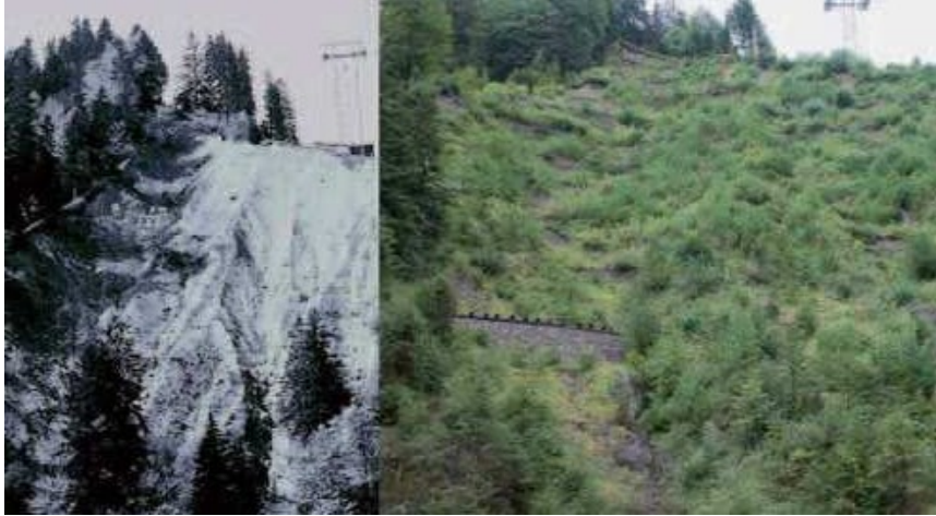
Figure 4.2 Schwandrübi scree slope (left) in 1978 before the application of gabions and hydroseeding, and (right) after the heavy rainstorm in August 2005 (source: left Forestry Service of Nidwalden; right WSL).
