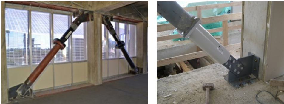
Figure 3.10: Example of visco-elastic dampers
