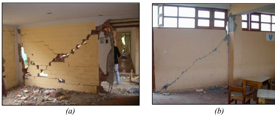
Figure 1.10: Example of a) interaction with the column; b) diagonal rod in infill wall
