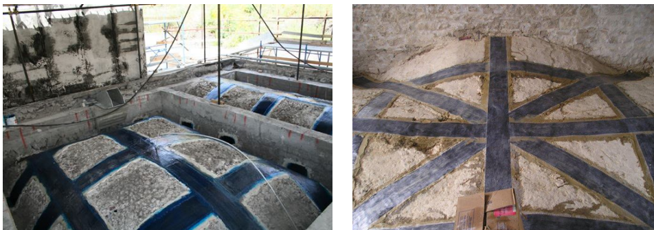
Figure 1.2. Interventions with FRP on masonry structures.
