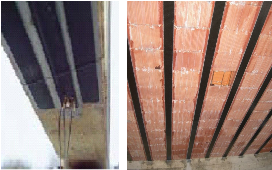
Figure 1.1. Interventions with FRP on reinforced concrete structures.
