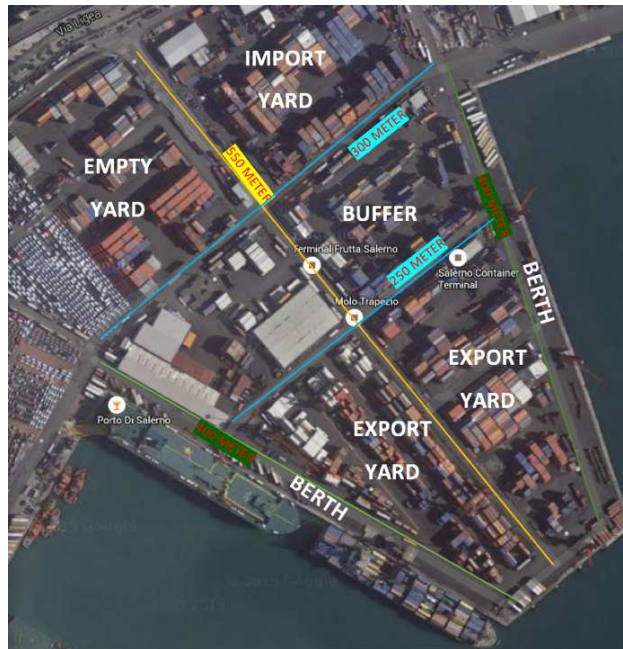
Figure 6.26 Aerial view of the port container terminal of Salerno (from Google Maps) with indication of the different yards and their dimensions.
