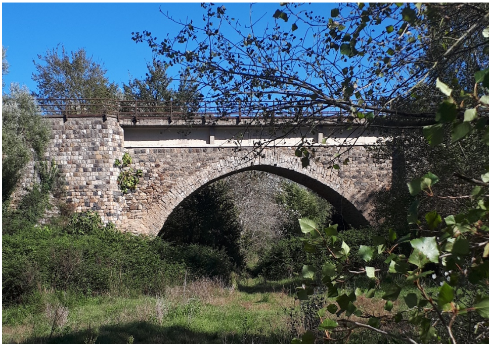
Figure 1: Masonry bridge “Pietra dell’Oglio”, 2nd century BC until, Monte Verde (AV).
