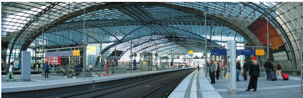
Figure 11: Hauptbahnhof Station in Berlin [126].
