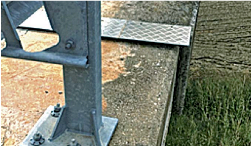
Figure 2.18: Relative displacement of the Abutment
