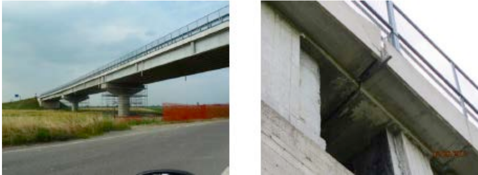
Figure 2.14: Precast concrete bridge outside Finale Emilia
