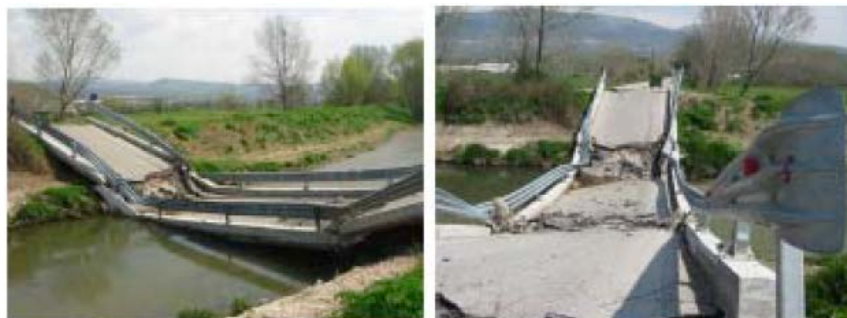
Figure 2.10: Bridge collapsed on the Aterno river, near Fossa (M. Indirli, 2010).
