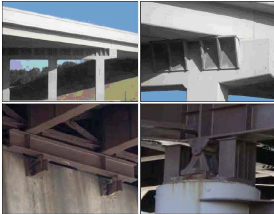
Figure 5.2: Example of an intervent of seat extender. (Wright, T 2011)
