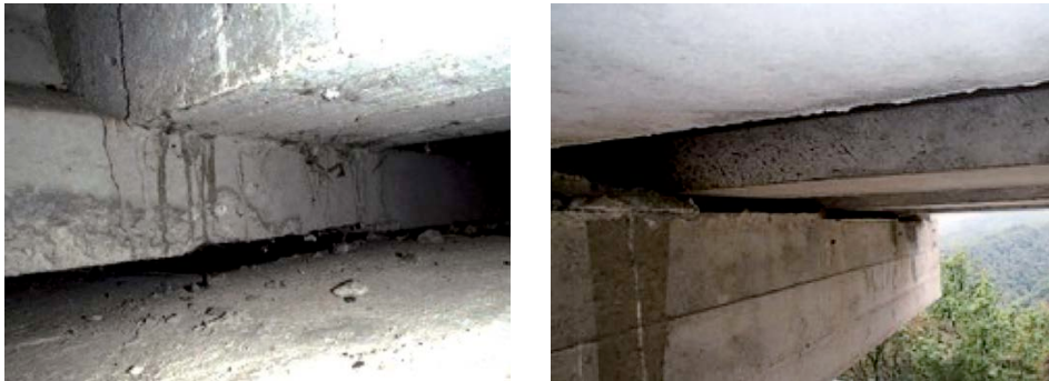
Figure 2.17: Elastomeric Bearing (Totaro photos).
