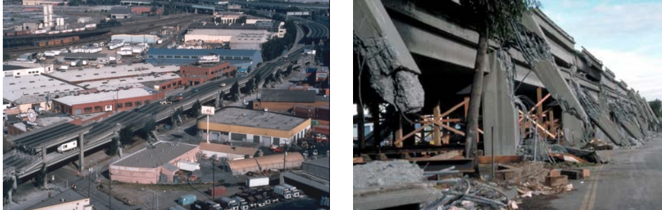
Figure 2.1: Cypress viaduct collapse left – aerial view; right – piers failure detailed view. (Nakata et al. 1999)
