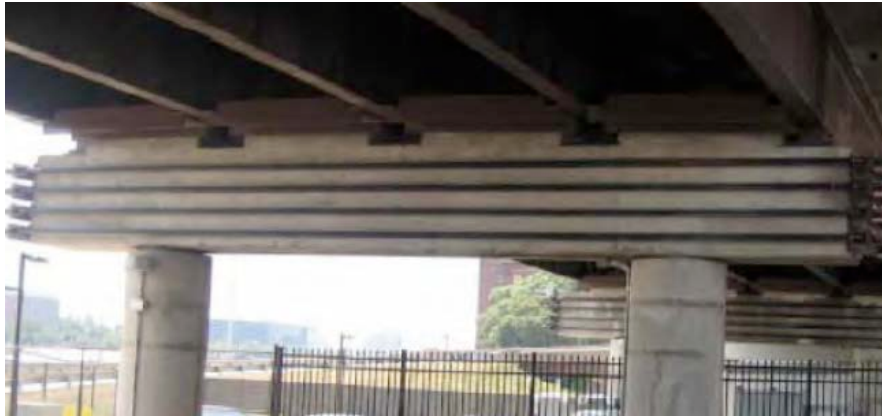
Figure 5.6: Prestressed cable for the retrofitting of the cap beam. (Wright, T 2011)
