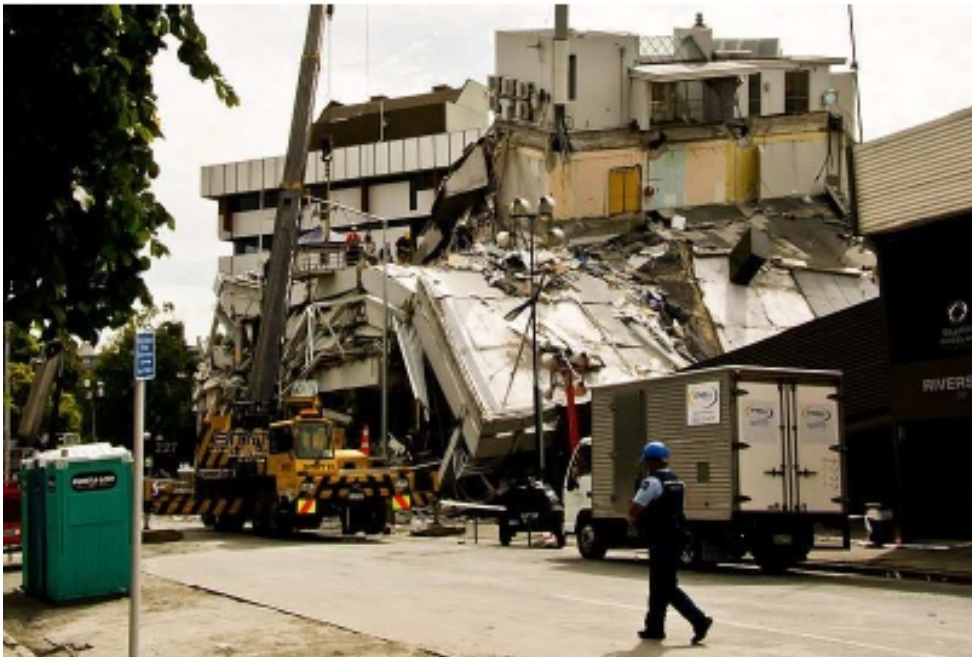
Figure 2.12: The Pyne Gould Corporation (PGC) Building following the 2011 Christchurch earthquake (Kam 2011).
