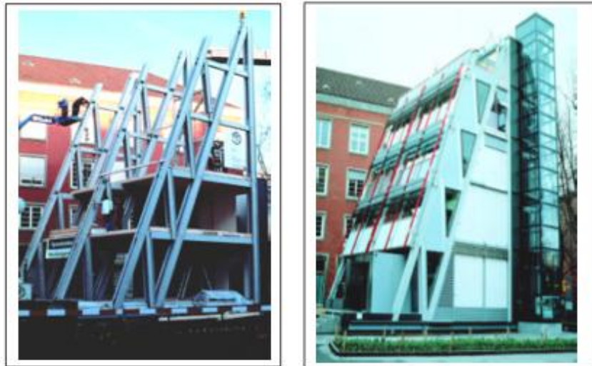
Figure 1.4. The All-Composite "Eyecatcher" Building in Switzerland.
