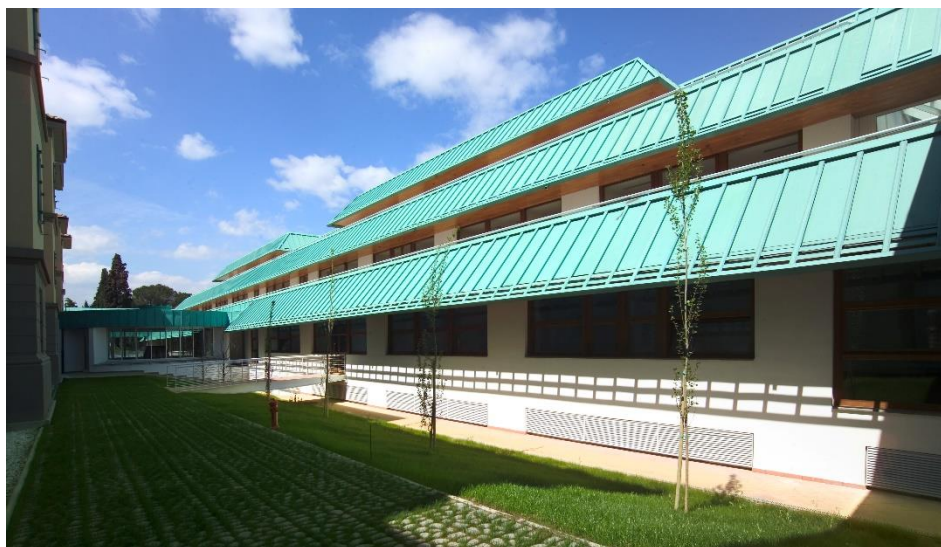
Fig. 3.29: Aggetti rivestiti in rame.
