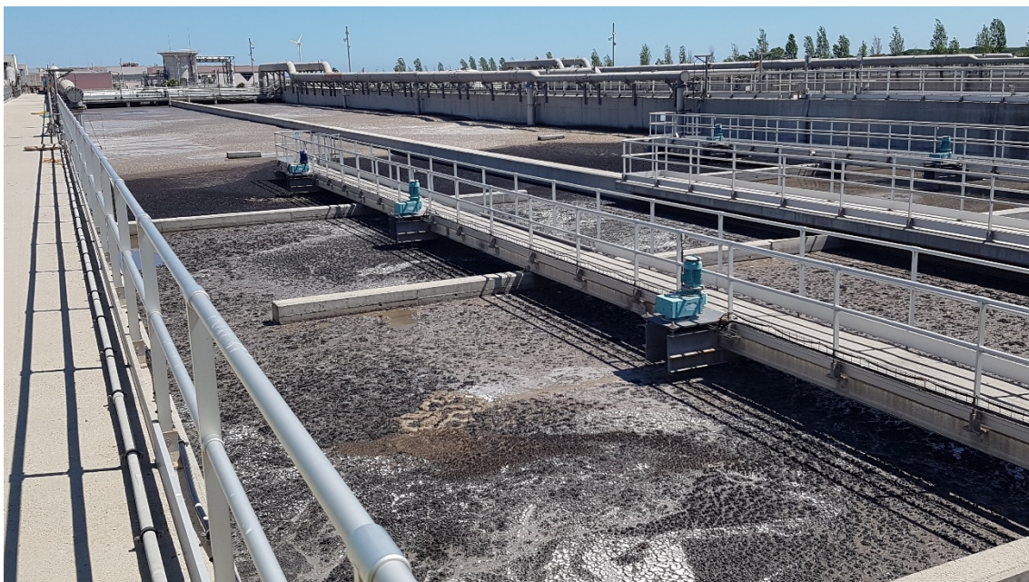
Figure 5 - Secondary treatment tanks at the Prat de Llobregat WWTP, Barcelona during and ANSWER-ITN visit. June 2016
