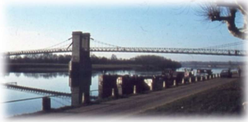
Retrofitting of the “Real Ferdinando” bridge (1990) Prof. F.M. Mazzolani
