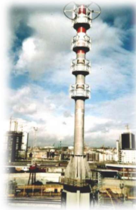
A tower for parabolic antennas
