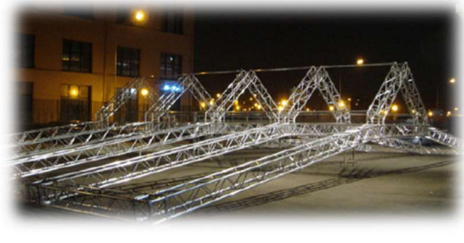
The Crystal (2012) Wilkinson Eyre Architects “The roof is made from recycled aluminium”
