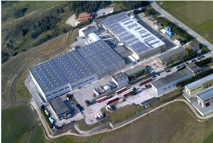
Figure 40: Image of the Lucart plant located in Avigliano.
