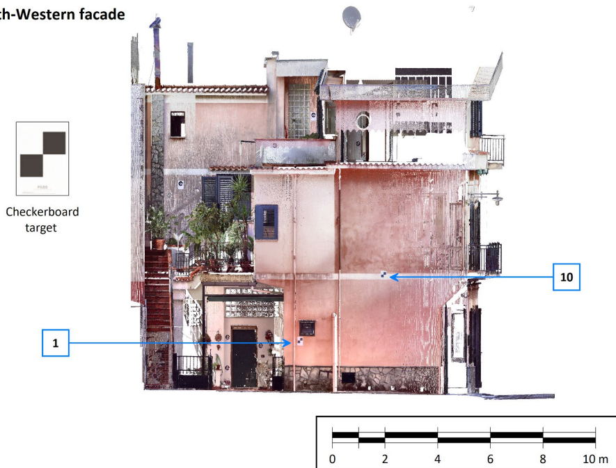
Fig. 2. 8. Distribution of the checkerboard targets on the South-Western facade.
