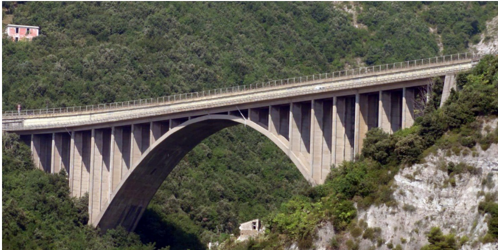
Figure 5.2 – View of the Olivieri Viaduct [220]
