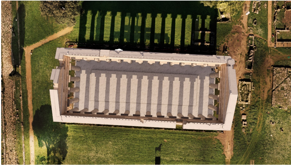
Figure 12.29 – Federated Revit projects rendered plan view representing the Temple of Neptune, its surroundings, and the monitoring seismometers network as of 2021 [AoE]
