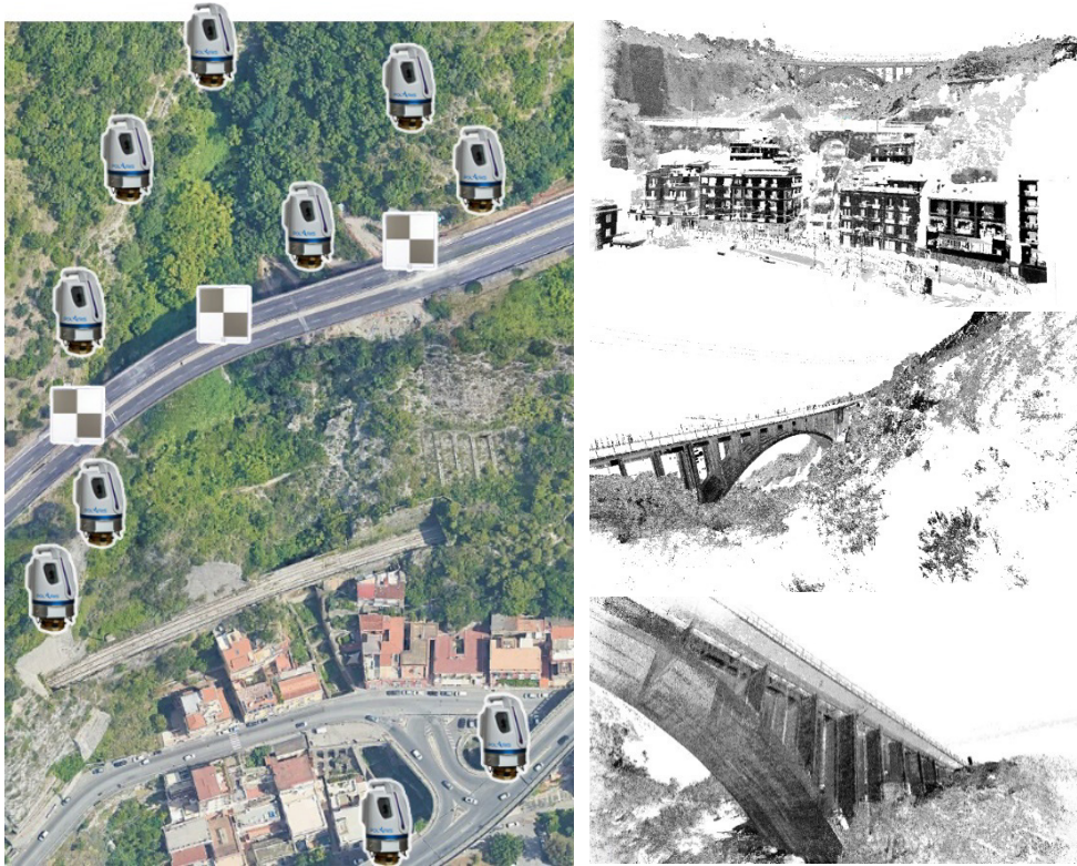
Figure 5.9 – Layout of the 10 surveying stations (left) and views of the aligned and georeferenced point cloud depicting the viaduct and the valley beneath (right) [222]
