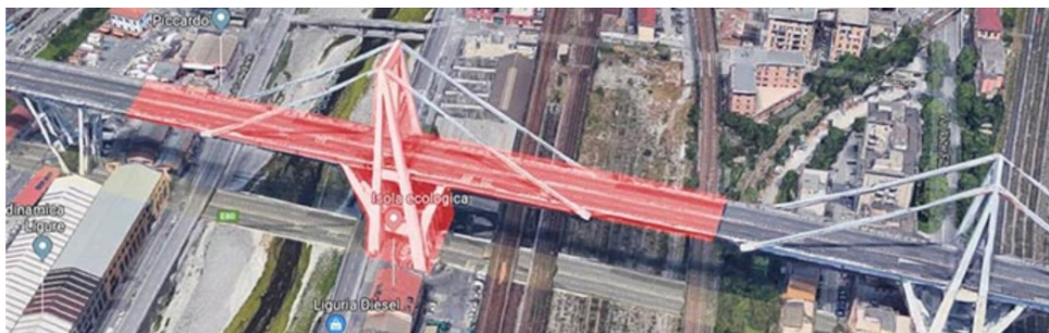
Figure 3.3 – Collapsed section of the Morandi Bridge [68]
