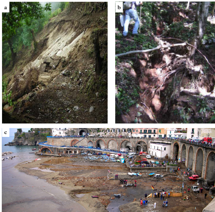
Figure 4.9 2010 event: a, b) slope instabilities in the upper part of the Dragone basin; c) damage at the outlet of the Dragone basin (photo from Autorità di Bacino Destra Sele , 2010).
