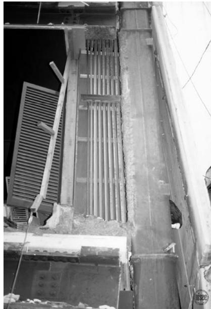
**Fig. 2.13** – Failure of beam-to-column fillet welded connection (Kobe Earthquake)
