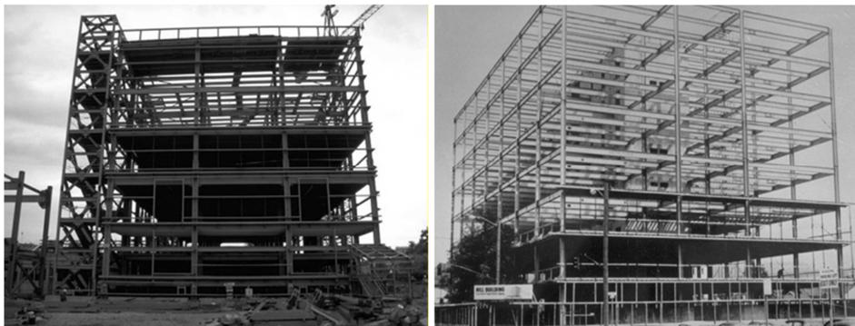
**Fig. 2.1 – Steel Moment Resisting Frames in U.S.A.**
