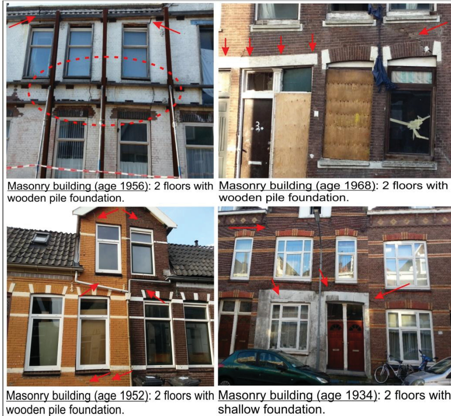
Figure 6.26 Some photos of damage recorded on the building facades during the field survey in Zaanstad and Dordrecht Municipality.
