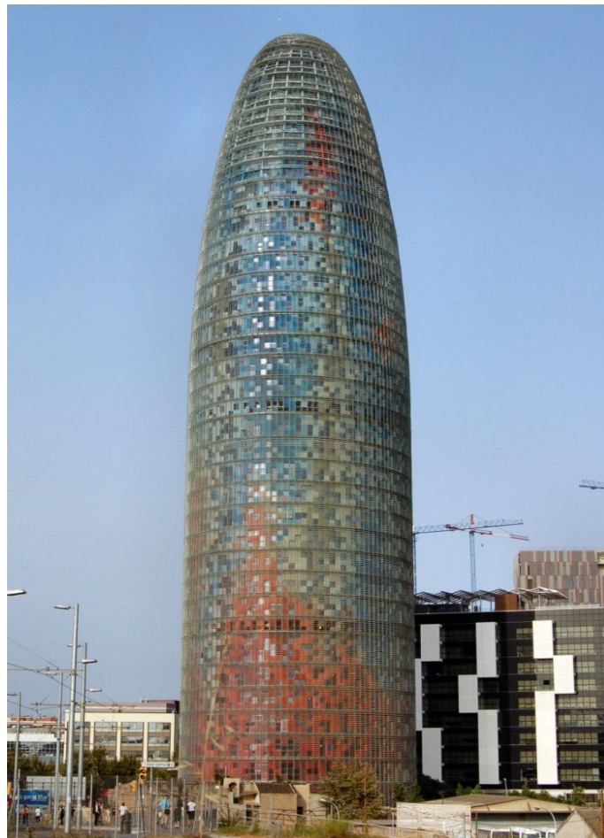
Fig. 1.15: Agbar Tower , Jean Nouvel - Barcellona, 2005.
