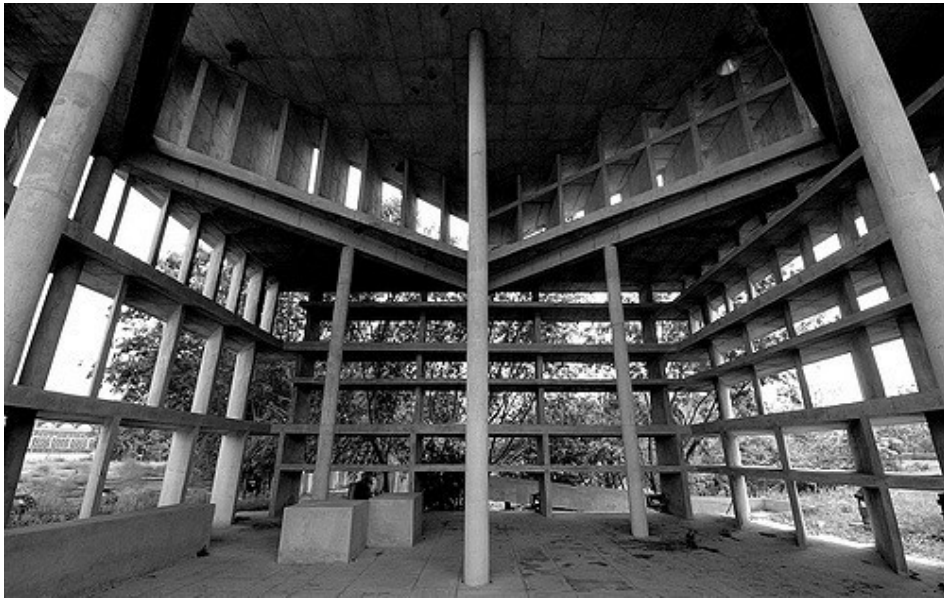
Fig. 1.8: Solar Pavilion , Le Corbusier - Chandigarh ,1965.
