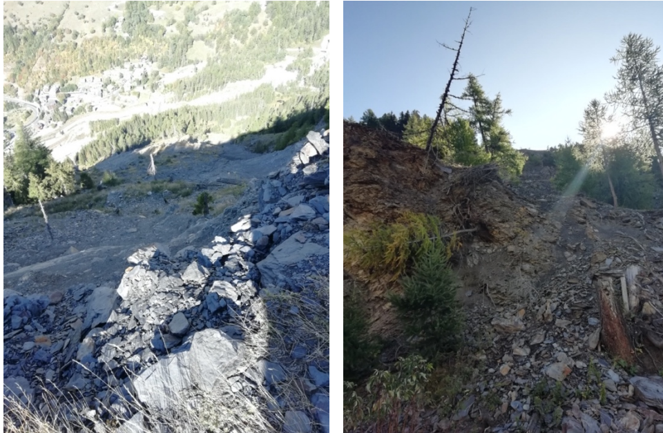
Figure 6.10: Details of the slope after instability events
