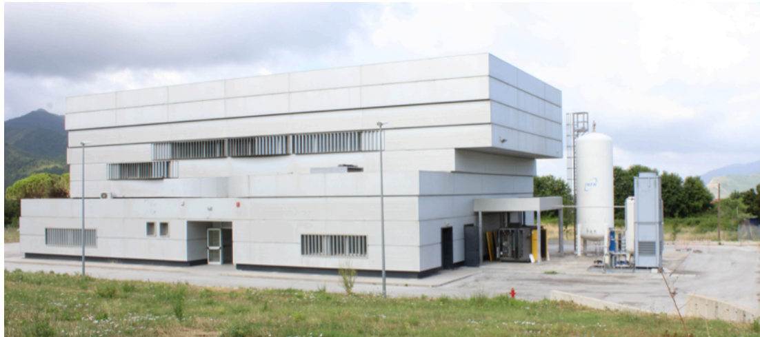
Fig.4.10 External view of the INFN Laboratory built on the University campus. On the right the water-cooling tower and the helium and nitrogen tanks. Besides the laboratory, there is also the 196 kW screw compressor.
