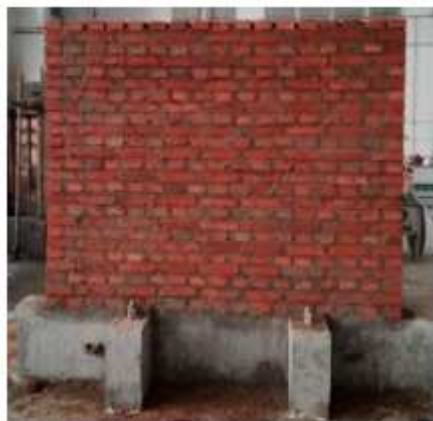
(a): Un-strengthened wall
