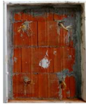
(b): Diatons placed inside holes + Application of liquid mortar
