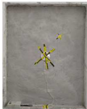
(d): Upgraded masonry wall
