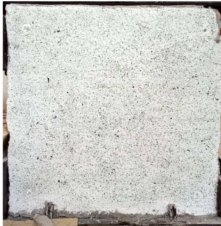
Fig. 9-4. Black spots/pattern surface of the wall specimen HBW5.
