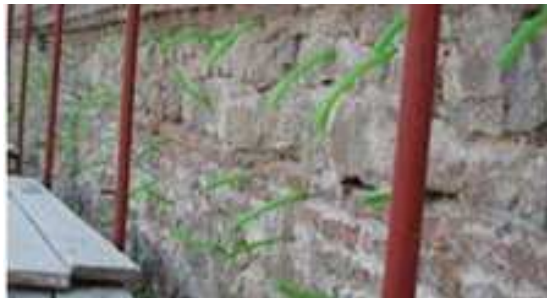
Fig. 2-17. Grouting (Christou and Elliotis 2016).
