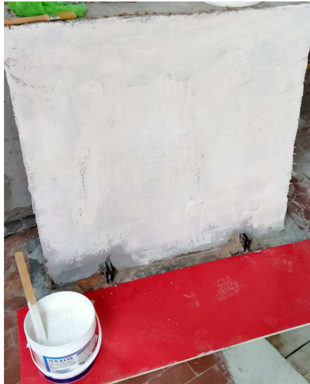
Fig. 9-2. Painting of masonry wall with white color.
