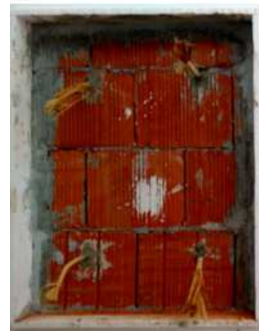
(b): Diatons placed inside holes + Application of liquid mortar
