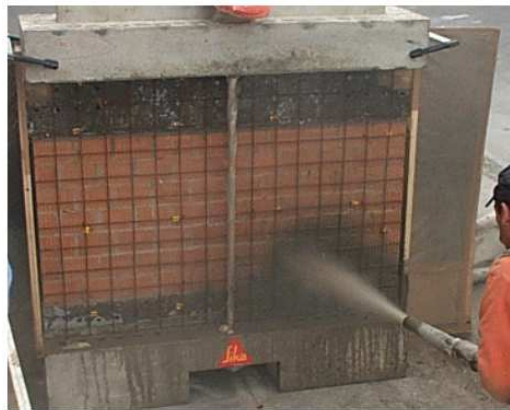
Fig. 2-14. Shotcrete spraying process (Wang et al 2018).
