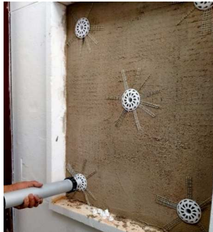
Fig. 2-20. Mortar injection in the diatons cavity.
