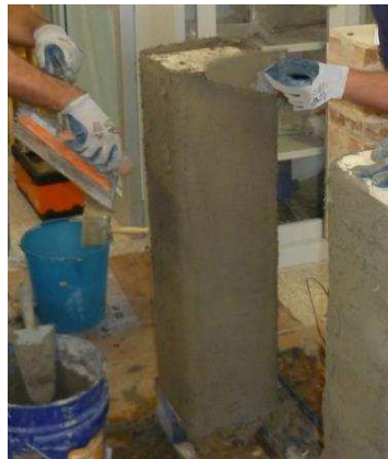
Fig. 2-27. BFRCM reinforcement (Fossetti and Minafò 2016).
