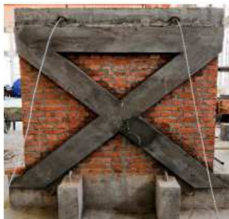
(c): strengthened wall
