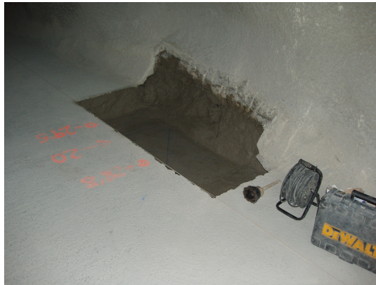
Figure 6.3: Excavation for the main plinth in Bypass 16.
