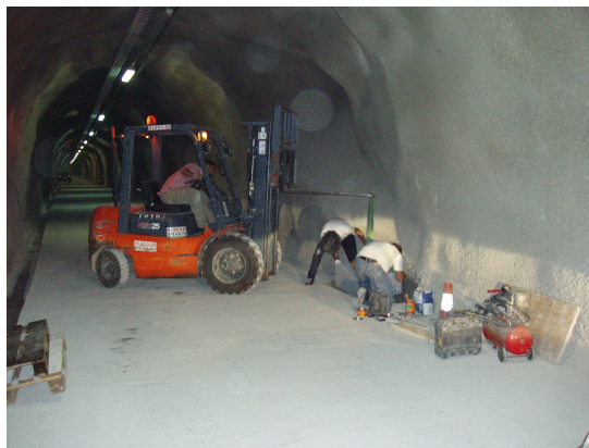
Figure 6.4: Positioning of the main plinth in Bypass 16.
