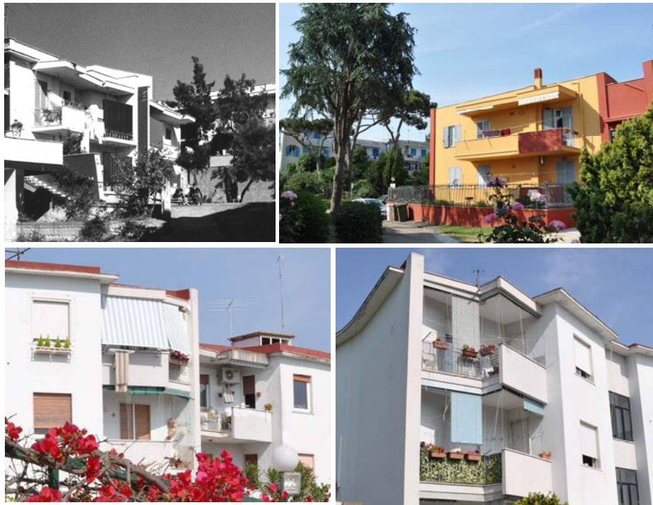
Fig. 5. 22: Different shading devices used. From the top left, the original brise soleil designed by Cosenza, Shade roll and venetian blind chosen by the users.
