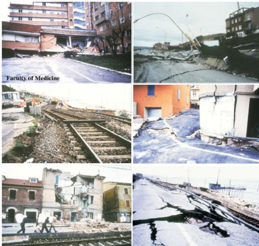
Figure 3.4 Ancona landslide: damage to man-made structures caused by the landslide (Cotecchia, 2006).
