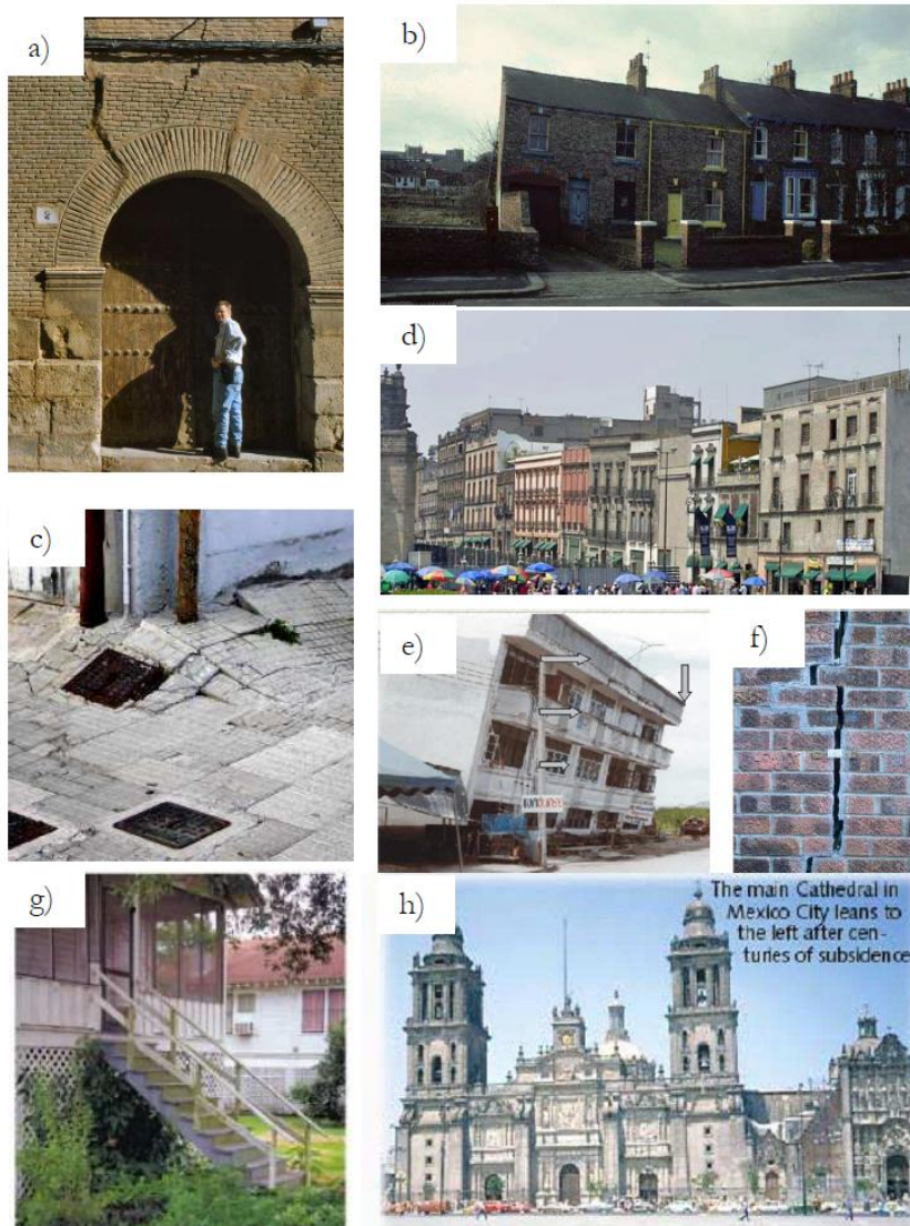
Figure 3.3 a) Hogging mode of failure with loss of support to the right of the picture Calatayud, Spain (Cooper, 1998); b) Sagging building damage Princess Road, Ripon (Cooper, 1998); c) Damage to road (Tivoli Terme, Italy) d) A row of buildings, showing effects of land subsidence (Credit: Chris Earle) e) settlement and titling of a building in Bangkok; f) An 18 mm crack in the wall of a house at Hutton Conyers near Ripon,UK (Cooper, 1998);g) building at the Everglades Experiment Station originally constructed at the land surface; latticework and stairs were added after substantial land subsidence ( http://water.usgs.gov ); h) damage to Cathedral in Mexico City.
