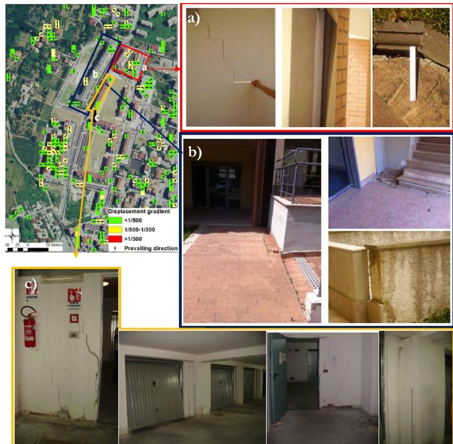
Figure 6.24 a) Map of displacement gradient and its prevailing direction, a)-c) occurred damages.
