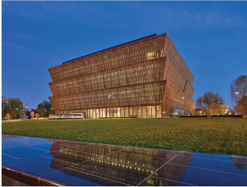
Figure 2: The three-tiered corona was inspired by West African Yoruba culture and art, the bronze-colored aluminum panels were modeled on ornamental ironwork made by slaves in Louisiana und South Carolina, and the main entrance serves as a reminder of porches used throughout the African diaspora. Copyright: Alan Karchmer/NMAAHC.
