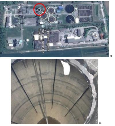
Fig. 5.1 - a) WWTP in Keszthely (Hungary). Red circle indicates the position of the digesters. b) Inner side of one of the digesters with the gas recirculation lances.
