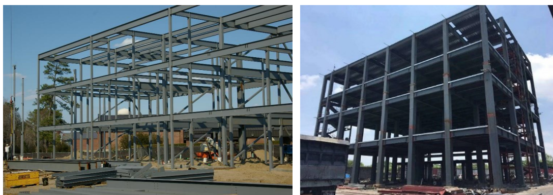
Figure 1.1 – Steel Moment Resisting Frames (MRFs)
