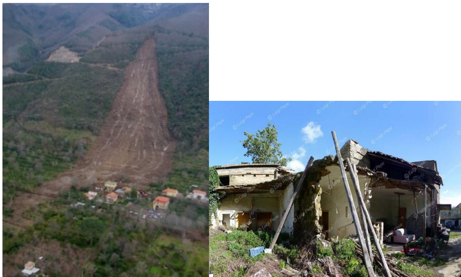
Figure 2-3. Example of a building destroyed by a debris avalanche occurred in the Nocera Inferiore area, Campania, southern Italy, 2005 (from Cascini et al., 2011).
