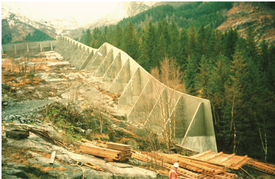
Figure 6-1. Example of concrete diverting dam at Odda, Norway (Barbolini et al., 2009)
