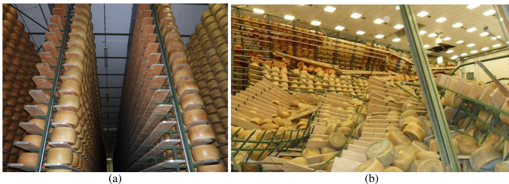
Figure 4.5: Typical storage system for Parmigiano cheese (a) and a collapsed one after something (b) (credits: Marco Simoncelli).
